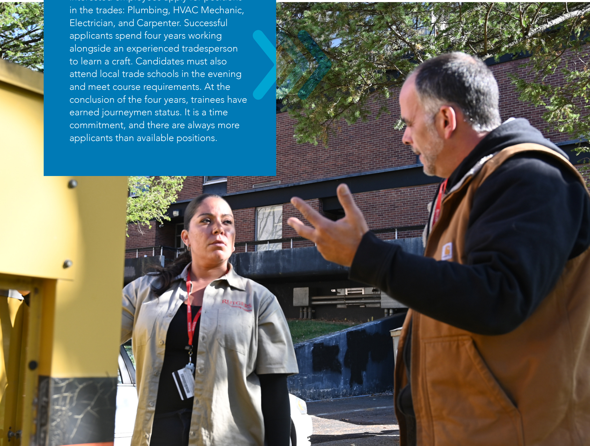
Electrician Jeff Manna shows Craft Trainee Sasha Alvarez how to maintain a generator on the Douglas Campus.
