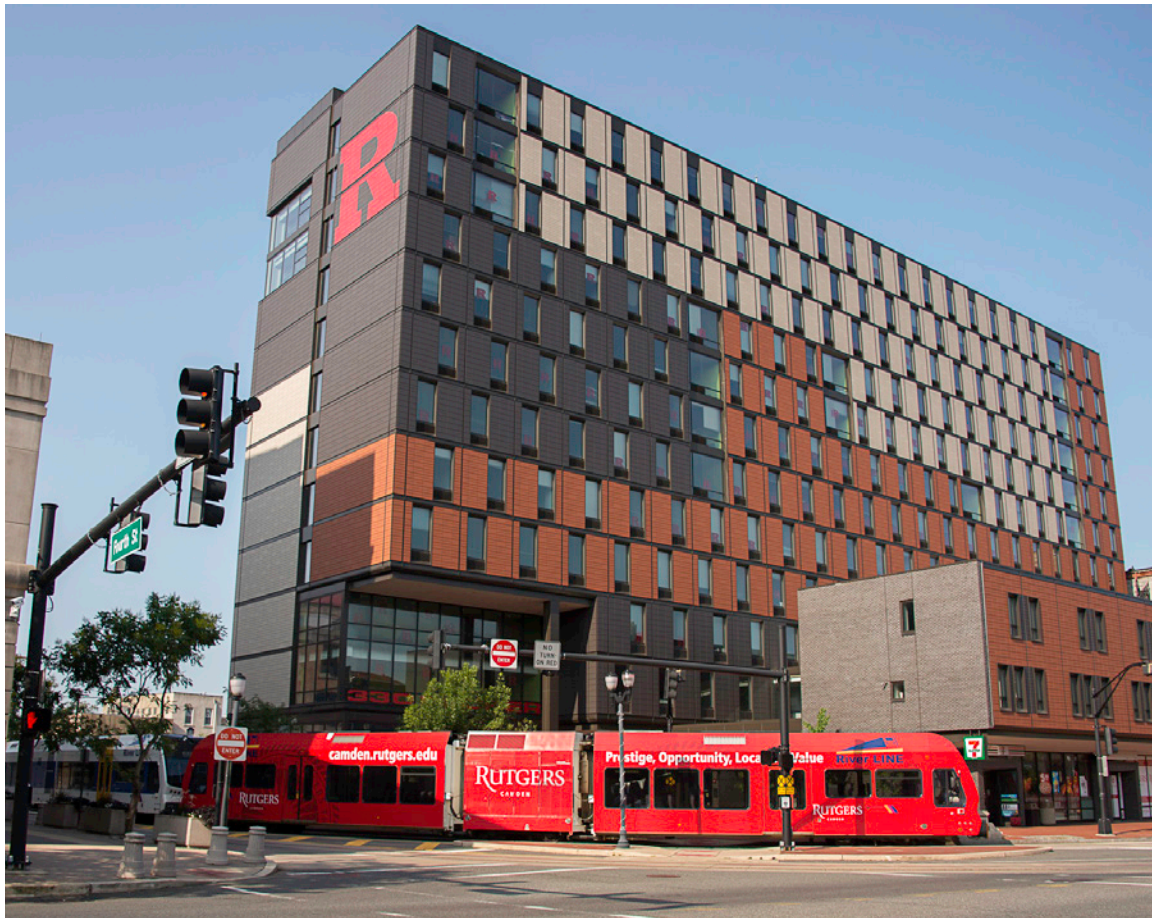
330 Cooper, new residence hall
