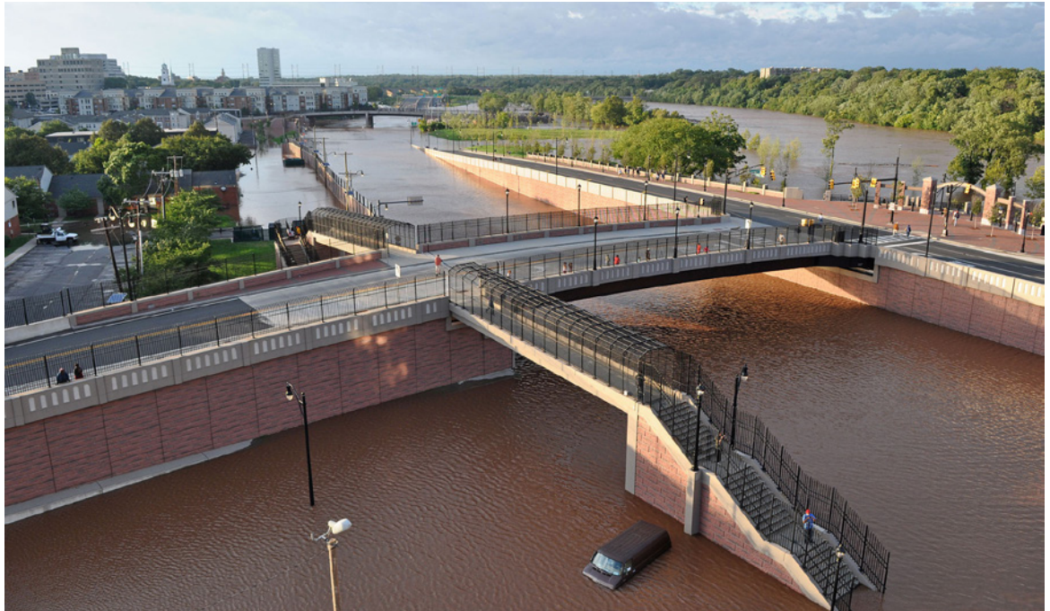
Flooding in New Brunswick after Tropical Storm Irene in 2011
